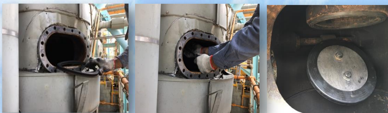
Flap Damper: Replacing New Packing
