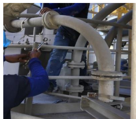
Installed Elbow Pipe with Ceramic Liner
