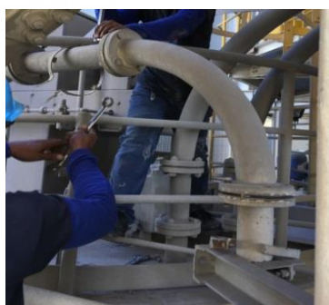
Installation of Elbow Pipe with Ceramic Liner
