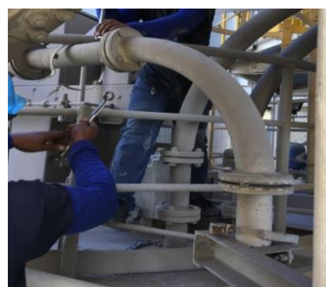
Installed Elbow Pipe with Ceramic Liner
