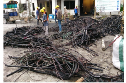
Burnt Control Panels and Wiring Cables removed from the Control Room
