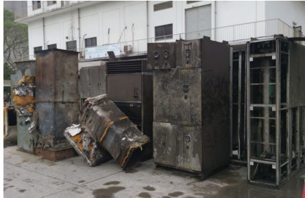
Burnt Control Panels and Wiring Cables removed from the Control Room
