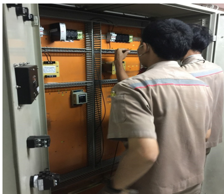
Installing Controller (As part of HFTR Installation)
