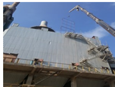
Lifting DE into ESP
