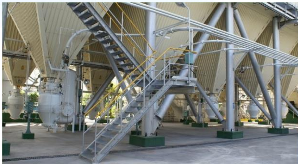
Ash Handling System in ESP
